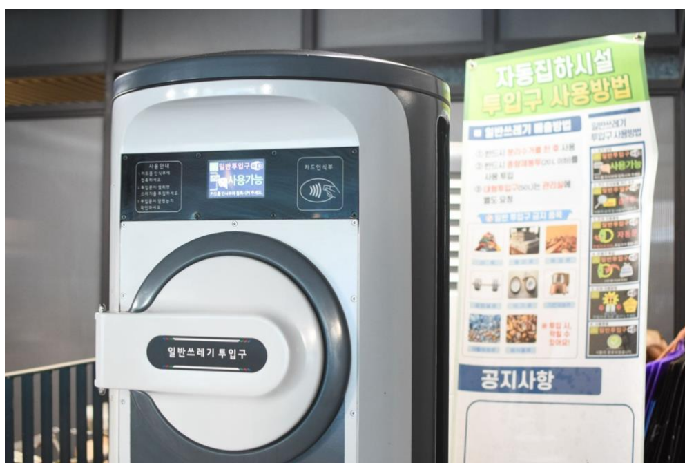
Figure 2: Envac's automatic waste collection system with disposal instructions
